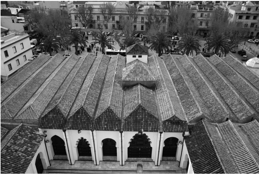
Figure 5. View of the roofs of the Great Mosque of Tlemcen (A. Almagro).
