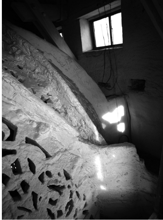
Figure 20. Detail of the extrados of the dome covering the maqṣūra in the supporting area of the ribs (A. Almagro).
